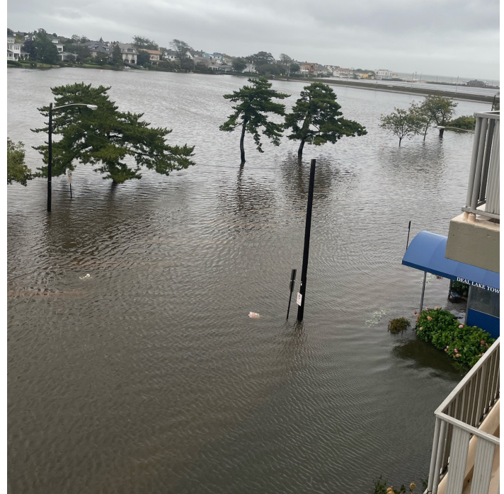
Flooding in Asbury Park and Loch Arbour, 2023
