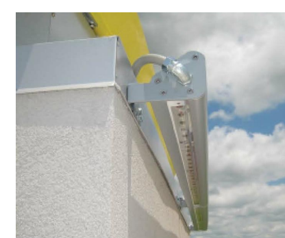
SECURITY LIGHTING HIRAF SERIES LINEAR LED FAÇADE LIGHT (LE2 & LE4) NOT TO SCALE
